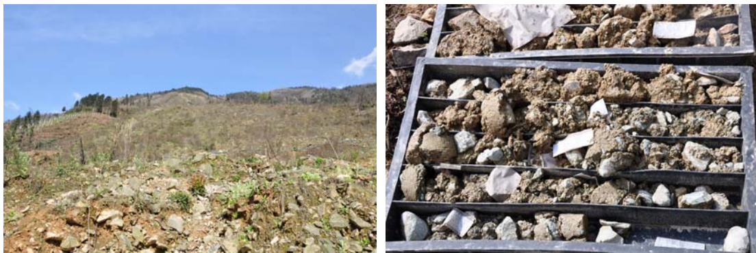
254 255 (a) Material on the landslide surface (b) Material in the shear zone
