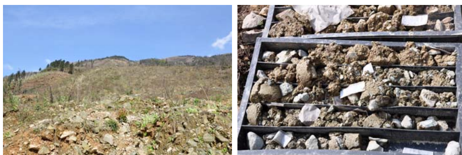
257 (a) Material on the landslide surface (b) Material in the shear zone
