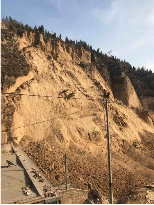
Figure 1. The cracking-sliding failure occurred in Shilou County of Shanxi Province on March 10, 2018 ( 110^{\circ}50'48.54''\text{E} , 36^{\circ}59'54.76''\text{N} ).
