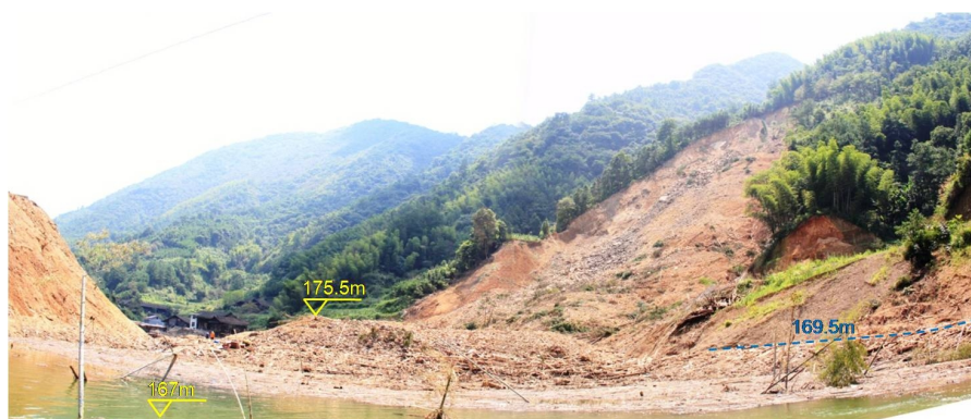
Fig. 7 Profile photo of Tangjiaxi Landslide, taken on July 23, 2014, when the water level is 167 m asl.
