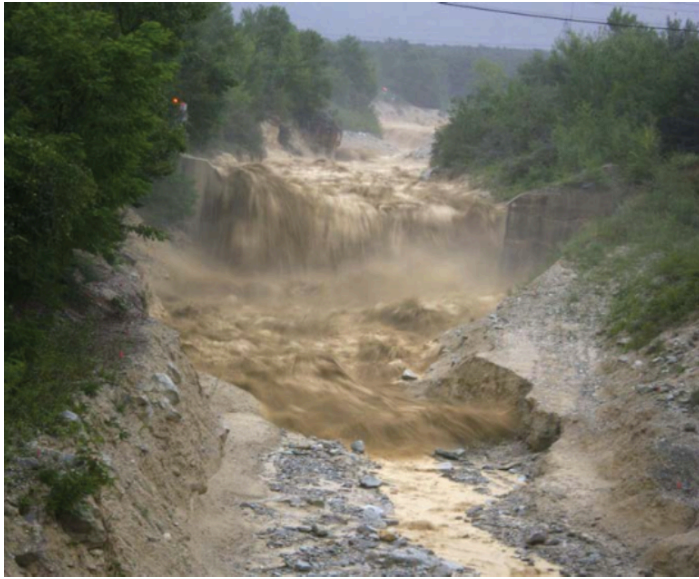
Figure 2: Photo of Illgraben debris flow event near Check Dam 28. Source: Brian McArdell, WSL.
