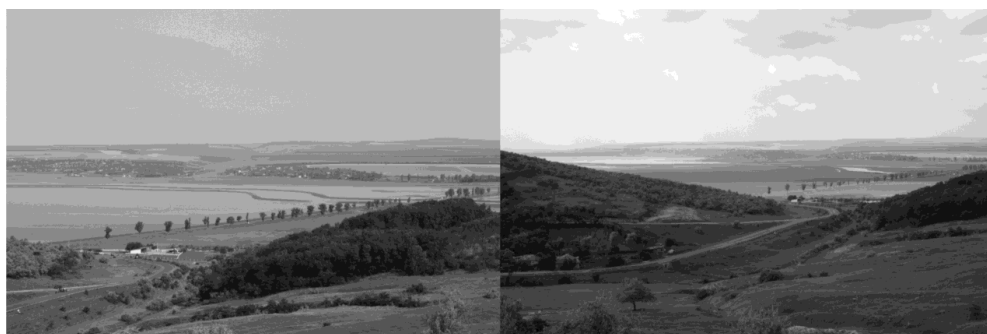
376 377 Figure 10. Polders on the Jijia and the floods recorded in the summer of 2010: storage of 378 excess water (left) and its elimination (right) 379
