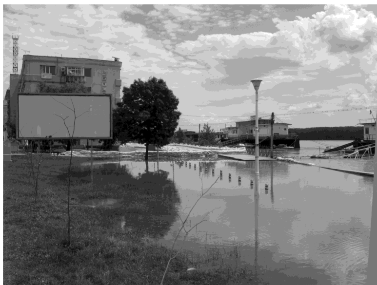
416 417 Figure 11. Flooding of the sea-cliff and the NAVROM headquarters in Galati 418
