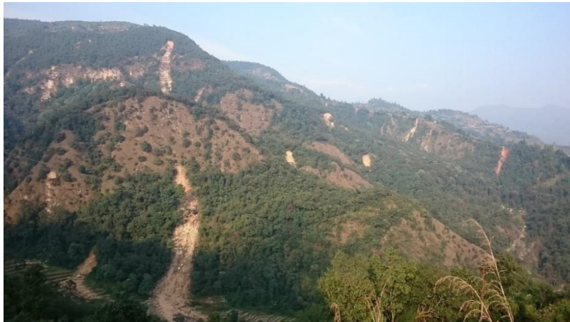
Figure 10: Photo of the area with so many several landslides near Pokhara watershed in Nepal
