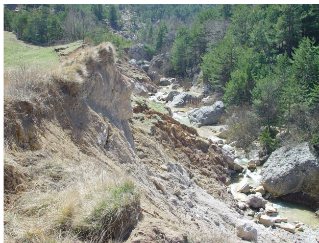
Figure 8. Picture of the landslide toe (taken on April 2003)
