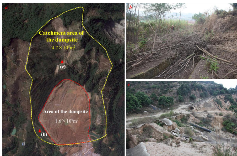
Fig. 6 a An overview of the catchment area (Google Earth image); b The surrounding peripheral drainage channel of the dumpsite was abandoned; c Damaged drainage pipes were not repaired and failed to divert surface run-off into the peripheral drainage channel. Surface run-off concentrated in the waste filling.
