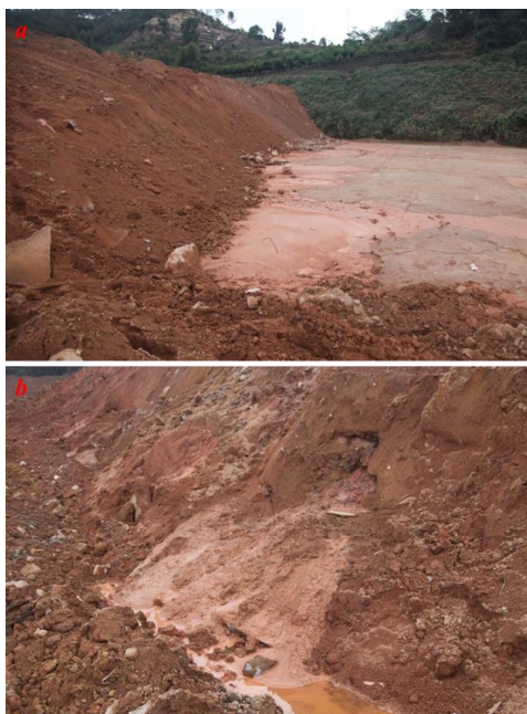
Fig. 27 Evidence of liquefaction near the opening of the failed retaining slope.
