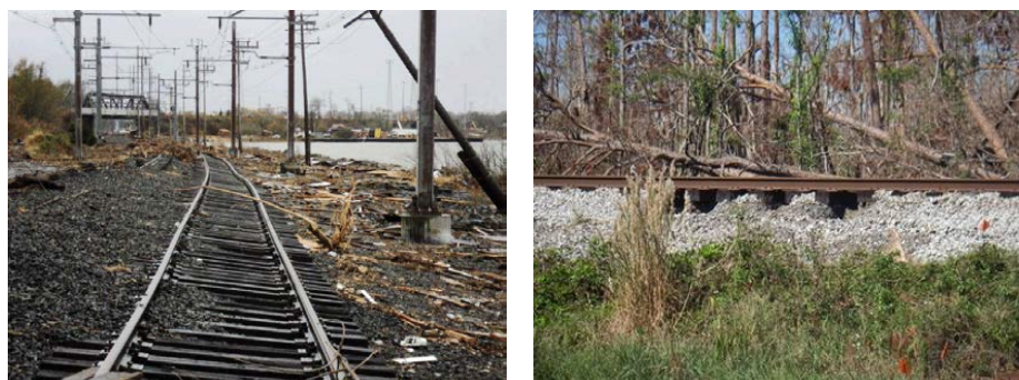
109 Figure 1 Railway embankment scour failures (left: New Jersey Transit tracks in New Jersey, USA after 110 Hurricane Sandy in 2012; right: CSX railroad tracks in Mississippi, USA after Hurricane Katrina in 2005)
