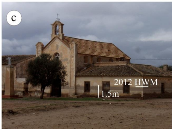
Figure 6. Pictures from the 2012 flood effects. A. Entrenchment of 2.5 m below Puerto Lumbreras Bridge. B. In-channel gravel quarry in Nogalte fan apex showing 4.5m channel entrenchment. C. Escucha chapel in Nogalte distal fan area showing the 1.5 m high water mark from 2012 event. D and E. Gravel mining impact on A-7 highway bridge after 2012 event; pillars are exposed in 2m. F. Headwards erosion due to gravel mining in the Béjar Rambla.
