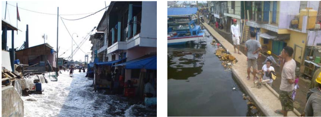
Figure 5: Pluit District in Jakarta is situated below sea level. The area suffered extensive inundation during a high tide on November 26, 2007 (Left). The thin dyke protecting the settlement was raised by about a meter after the 2007 event by the local government, obstructing people's vision of the sea. The photo was taken on October 18, 2013 (Right). (Photos: courtesy of Brinkman J.J., Deltares).
