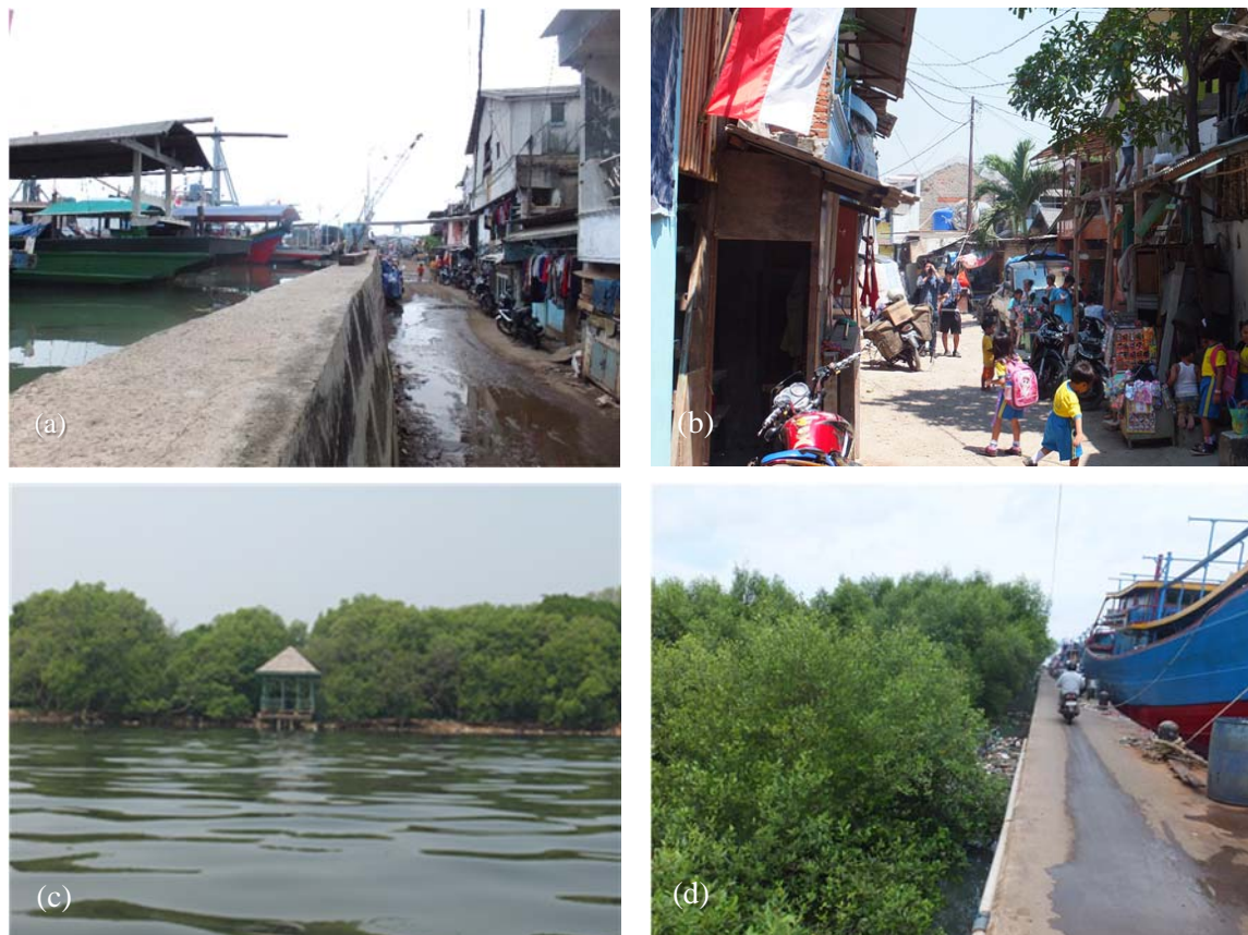
5 Figure 2: Coastal areas around Jakarta (photos taken by the authors during field surveys in the period between May 2015 and February 2016) (a) A thin coastal dyke protecting a community experiencing rapid subsidence (Pluit District, northern Jakarta). Leakage of seawater through a concrete joint was observed during the authors' visual inspection on February 6, 2016. The sea level was 1.3 m higher than the road. (b) The town center of Pluit, with a high population density and long narrow paths. (c) Mangrove conservation site in Jakarta (see Fig. 3 on its location) (d) Mangrove rehabilitation site in the Jakarta Fishing Port (see Fig. 3 on its location). The mangrove belt is around 20 m thick and can effectively protect the port basin from wind waves.
