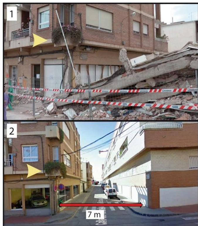
381 382 Figure 5 An example of the maximum impact distance evaluation. Photographs by : 1 Marc 383 Bertran Rojo, 2 (Google Street).
