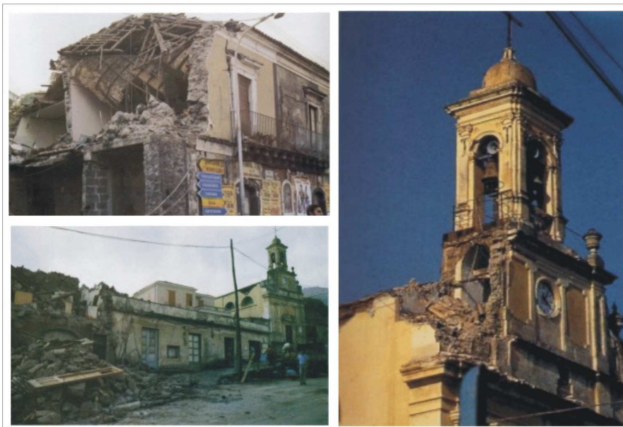
Fig. 3. Photos of damage caused during the 25 th October earthquake at Fleri village ( http://www.ct.ingv.it/macro/etna/html_index.php ).
