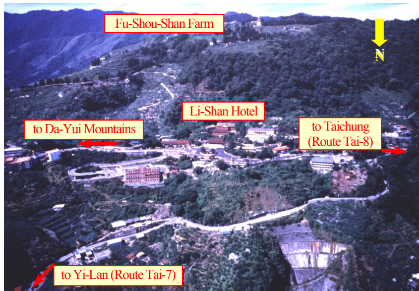
Fig. 1 Overlook Li-Shan landslide area northward from Fu-Shou-Shan Farm at the upslope
