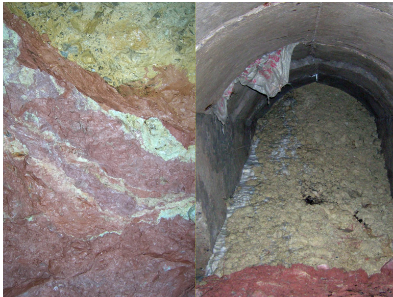
Figure 17. The sliding zone and slip mass in tunnel near by the eastern lateral edge.
