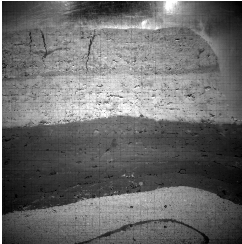
Figure 29. Tension cracking in trailing edge and top.
