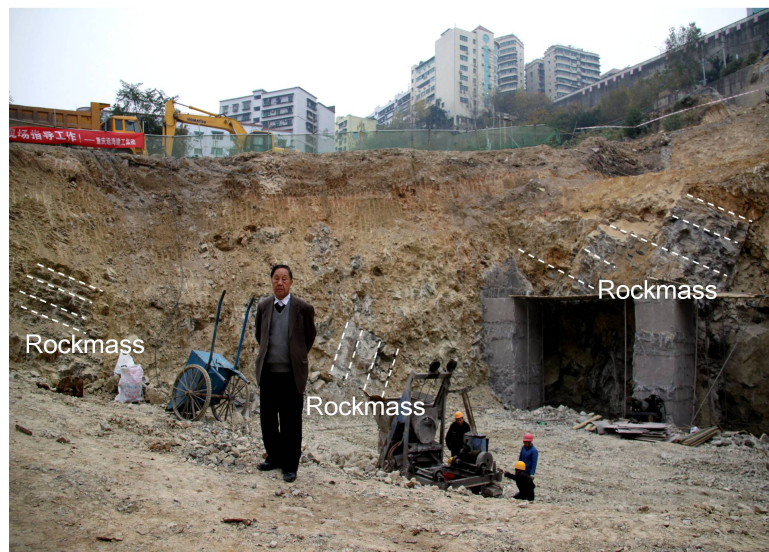
Figure 25. Rockmass showing their anomalous attitudes each other in the western wall of the foundation pit, and this kind of geologic structure is only generated by landslides.
