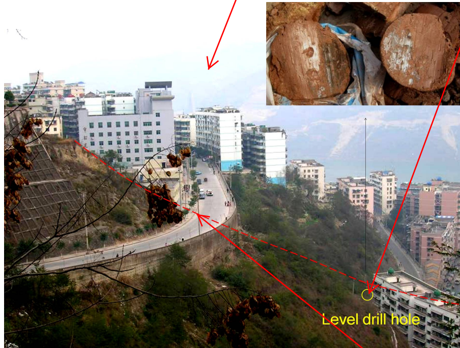
Figure 19. The sliding scrape in level drill hole near by the western lateral edge.
