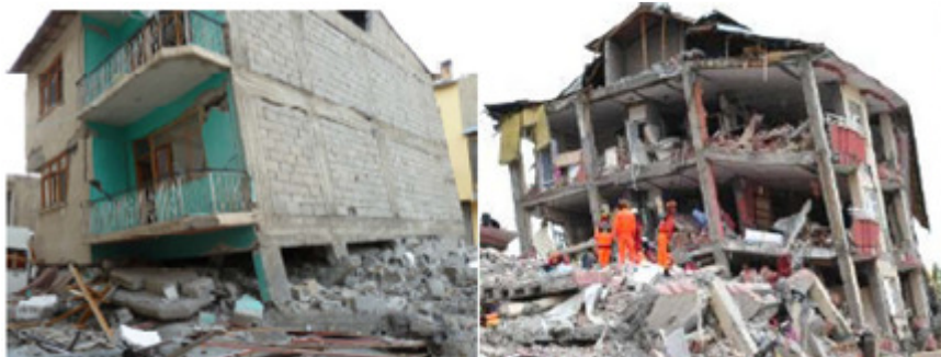
Figure 22. Damage observed in buildings with insufficient lateral rigidity.
