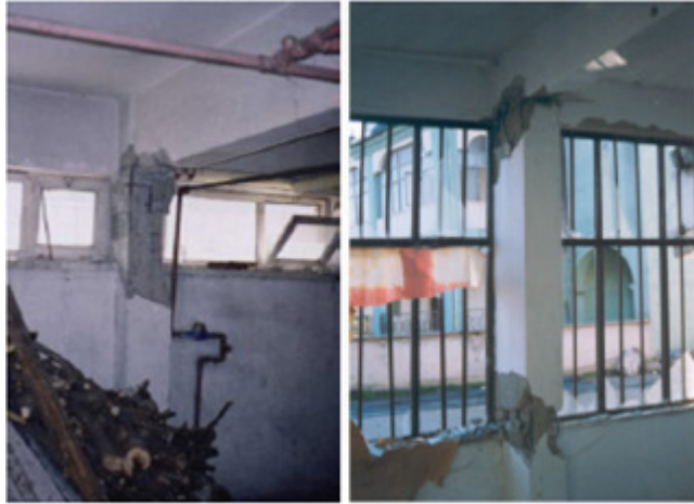
Figure 11. Short column formation caused by ribbon windows [8].
