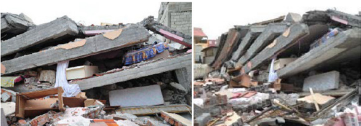
Figure 20. Full collapse of a building as a result of plastic hinges in the bottom and top zones of columns in a reinforced concrete structure in Van-Ercis [1].
