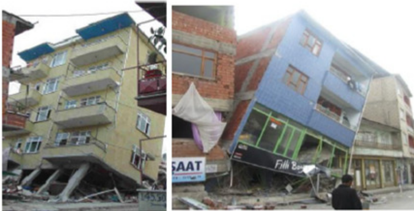
Figure 12. Examples of damage related to soft-story and weak story irregularities (Source: Ahmet Topçu).
