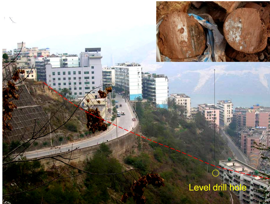
Figure 19. The sliding scarp in level drill hole near by the western lateral edge.
