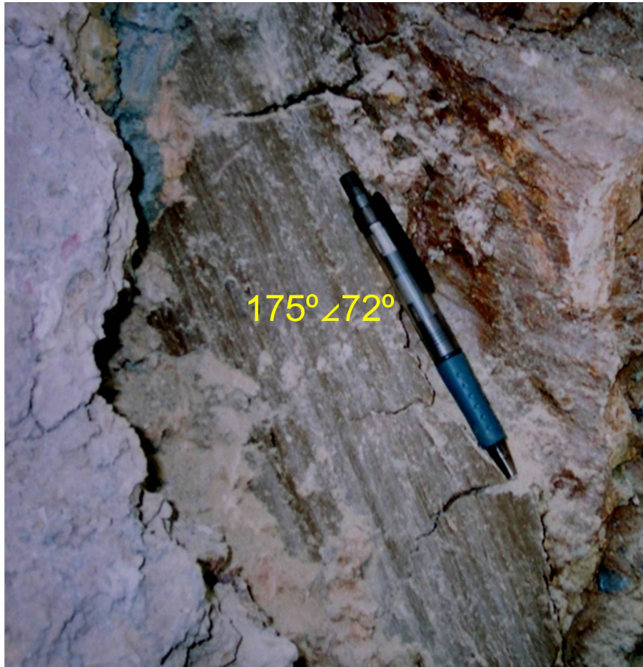
Figure 15. The sliding scarp of the scarp be revealed by foundation excavation.
