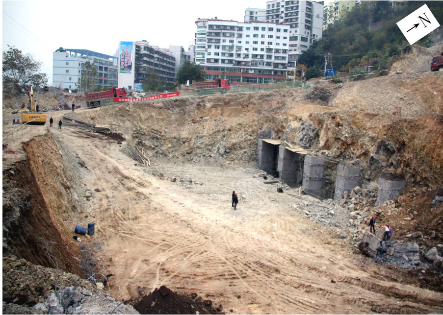
Figure 22. Overview of the foundation pit (photograph taken in 2013).
