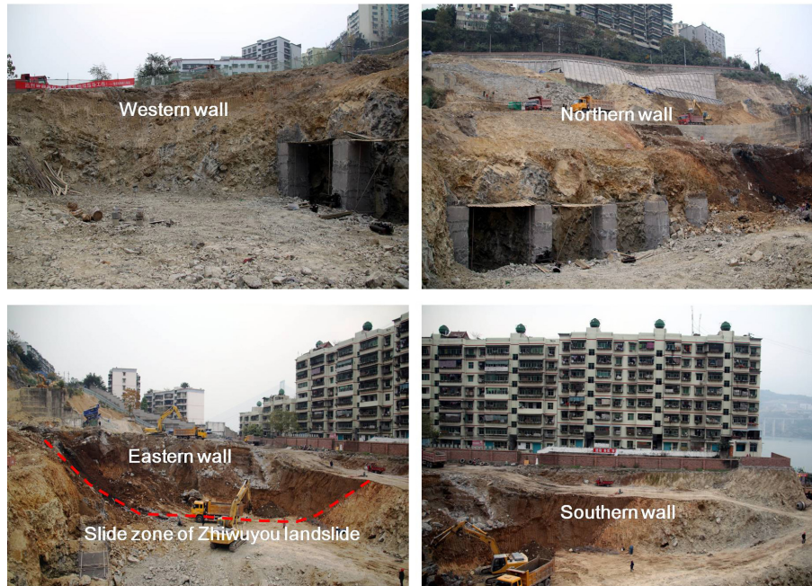
Figure 23. The geologic structure of four walls in the foundation pit.
