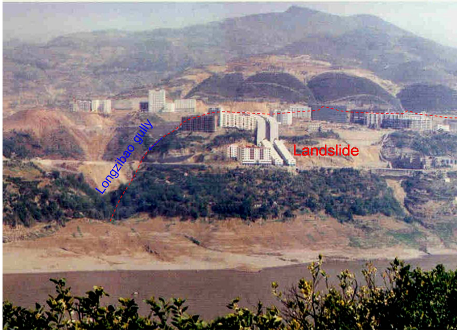
Figure 18. The western lateral edge of the Sanmashan landslide.
