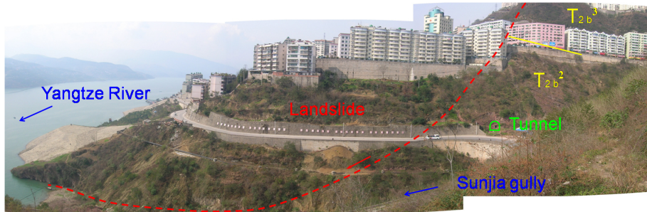
Figure 16. The eastern lateral edge of the Sanmashan landslide.
