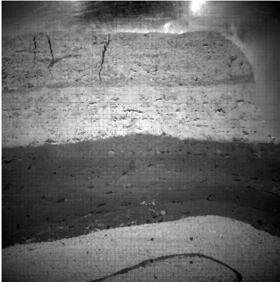
Figure 29. Tension cracking in trailing edge and top.
