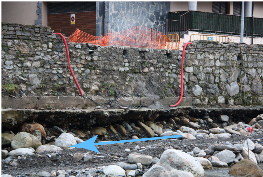
Figure 13. Vertical incision in a channelization at Les. Imbricated clasts below the scoured dyke prove that the Garona River entrenched into its channel bed deposits. The flow direction is indicated with a blue arrow (photo Glòria Furdada, 15 January 2014).
