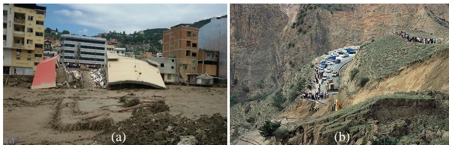
Figure 1. (a) Building collapse at Zirab in Mazandaran province and (b) landslides on the Chalus road due to heavy rainfall.
