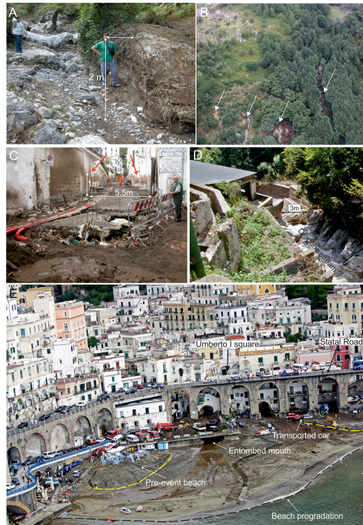
Figure 5. Geo-environmental effects induced by the 9 September 2010 rainstorm in the Dragone catchment. (a) Linear erosion engraving tributary channel. (b) Soil slip (arrows) at P. Castagne. Location in Fig. 3a. (c) Partial outbreak of the main road (Via dei Dogi) in the Atrani village. Red arrows indicate maximum height of the flow reaching ca 1 m above the street pavement. Location in Fig. 13. (d) Site of temporary damming in correspondence of a man-made structure built in the stream bed. (e) Terminal fan at mouth of the Dragone stream.
