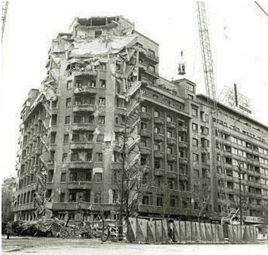
Figure 8. Wilson block of flats after earthquake (1977). Source: courtesy of Rezistență urbană.
