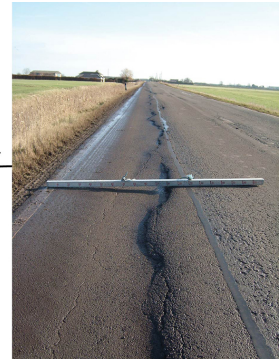
Figure 2. Soil processes leading to longitudinal cracking of road surface with photo example from Fodderdyke, Lincolnshire (photograph: Lincolnshire County Council, reproduced with permission).
