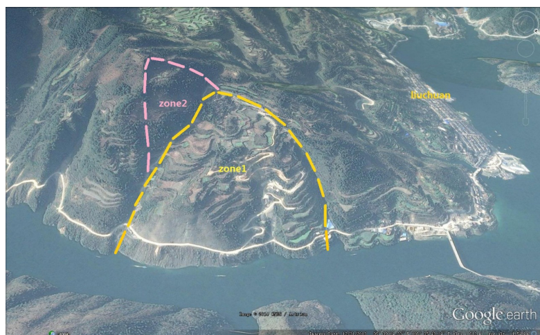
Figure 2. The Donglingxin landslide facing the Qingshui River (taken form Google earth).
