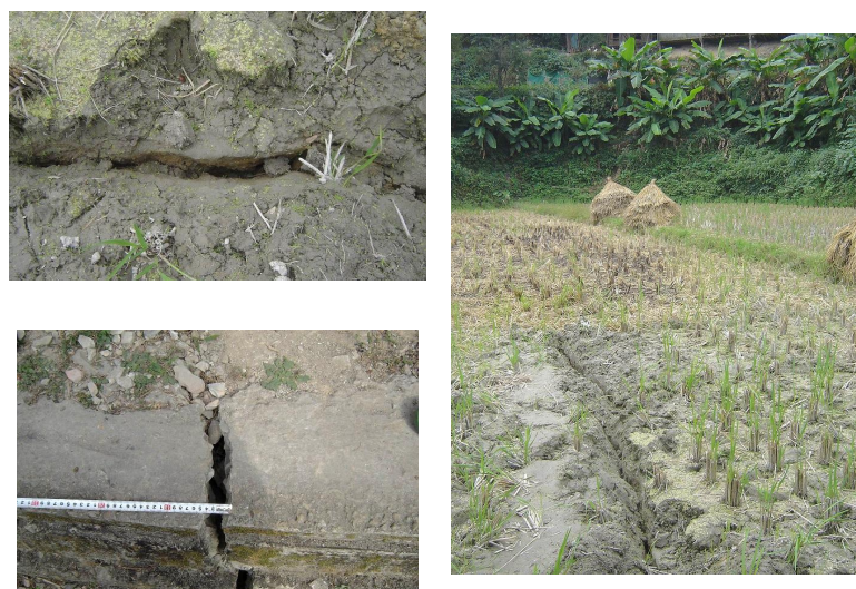
Figure 6. Photo of cracks in farmland at elevation 692 m.
