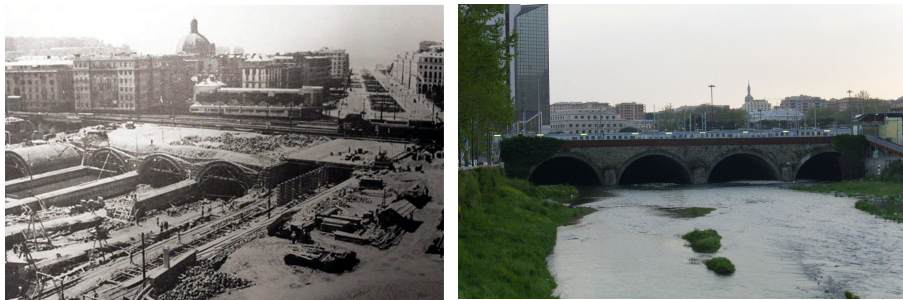
Figure 10. The Bisagno stream culvert during its construction (1930) and nowadays.
