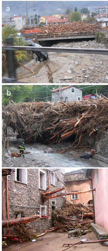
**Figure 1.** LW clogging in the Magra river catchment after the 2011 flash flood. **(a)** Upstream view of a bridge in the town of Brugnato. Note also the evident sediment deposition below the bridge; **(b)** downstream view of a huge wood jam trapped by a bridge in the village of Pignone; **(c)** street clogged by LW in town of Borghetto Vara. Source: Autorità di Bacino del Fiume Magra and Provincia di La Spezia.
