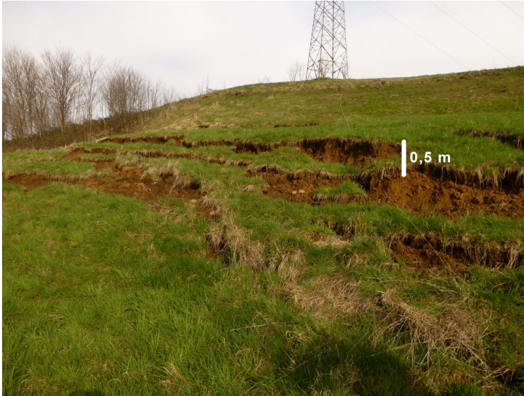
Figure 5. Main scarp of Carrè landslide.
