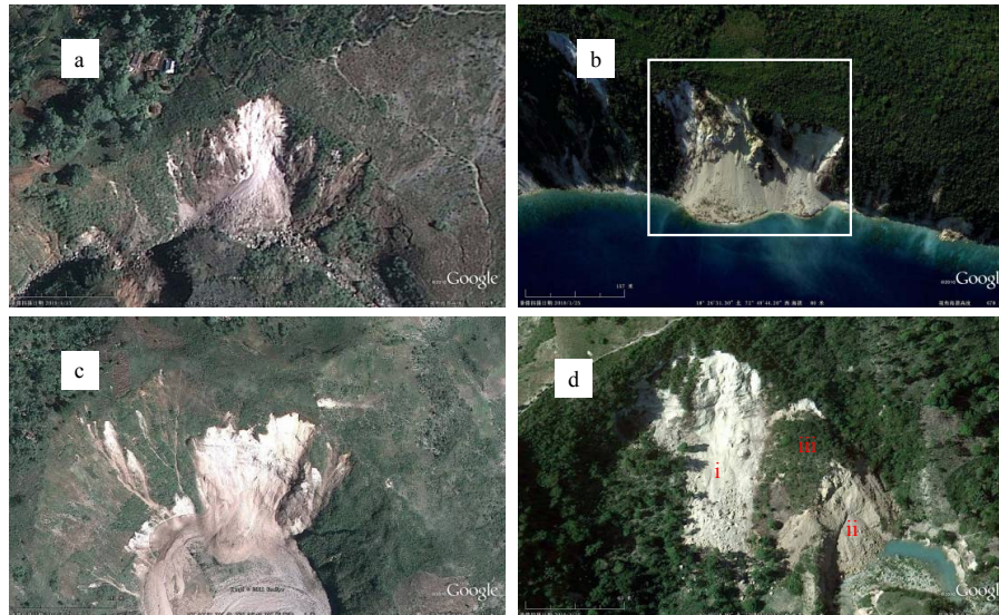
Fig. 8. (a) and (b) are two rock falls occurred at ( 18^{\circ}28'07.75'' N, 72^{\circ}29'15.00'' W) and ( 18^{\circ}26'31.30'' N, 72^{\circ}49'44.20'' W), respectively. (a) was taken on 13 January 2010 (upward is northeast) and (b) was taken on 25 January 2010 (upward is south). (c) is located at 18^{\circ}28'51.78'' N, 72^{\circ}26'42.00'' W, taken on 13 January 2010 and upward is north. (d) shows several rock falls at 18^{\circ}19'38.90'' N, 72^{\circ}40'01.32'' W, and the images was taken on 25 January 2010 (upward is west).
