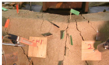
(e) Cracks developed at slope surface and crest originated from the loading plate
