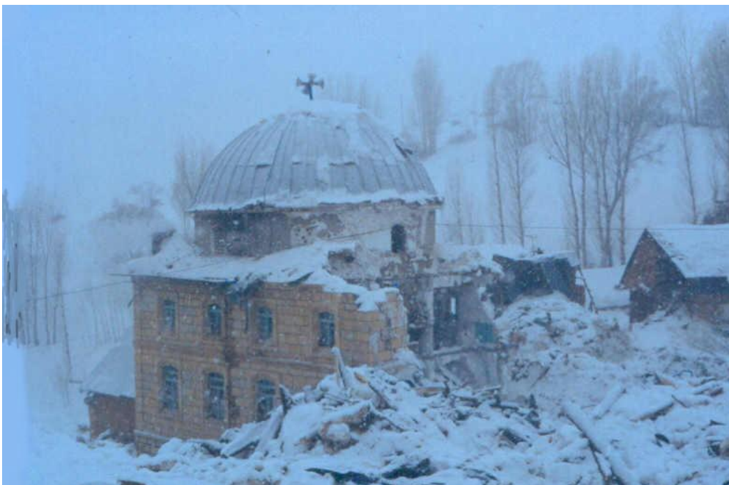
Fig. 4. Destroyed mosque due to 1993 avalanche event in Üzengili village.
