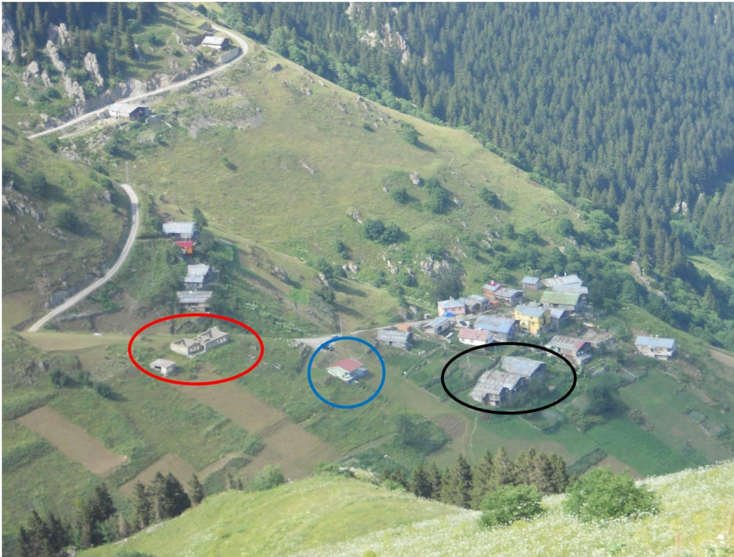
Fig. 5. Damaged school building (red ellipse) and houses (black ellipse) due to the 1981 – house indicated in blue circle constructed in 2004.
