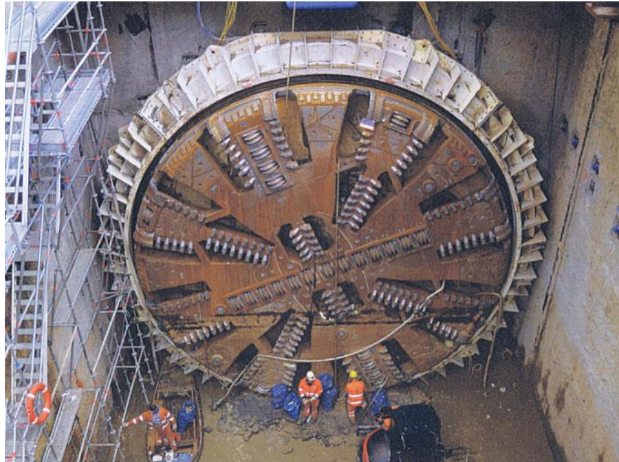
Figure 2. Shield machine TBM arriving in the target shaft (Mark et al., 2012).
