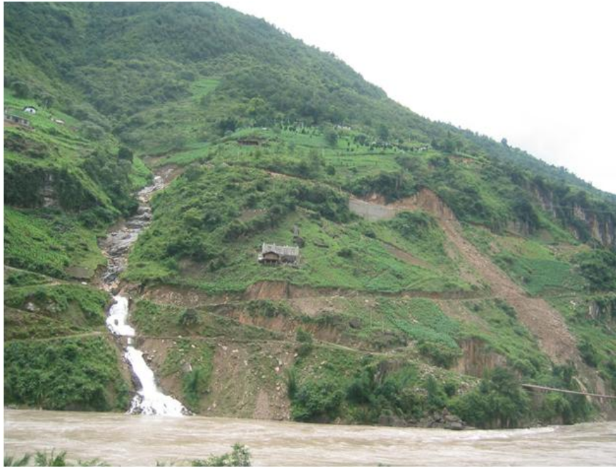
Figure 3. Road leading to a mountain village on the west side of the Salween River about 45 km south of Fugong. Upper portion of the road had (SFG1) the lowest landslide erosion of all surveyed segments, while the lower portion of the road (SFG2) had fewer numbers of, but larger, cutslope failures. Landslide erosion rates were significantly higher at SFG2 compared to SFG1 – 3.5 times higher for fillslope and 4.4 times higher for cutslope failures. Access bridge across the river is in the lower right corner of the photo.
