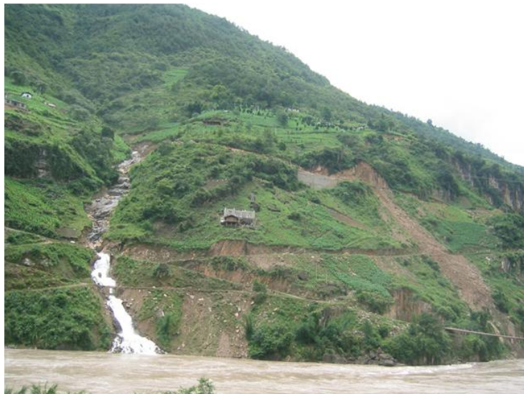
Figure 3. Road leading to a mountain village on the west side of the Salween River about 45 km south of Fugong. Upper portion of the road had (SFG1) the lowest landslide erosion of all surveyed segments, while the lower portion of the road (SFG2) had fewer numbers of, but larger, cutslope failures. Landslide erosion rates were significantly higher at SFG2 compared to SFG1 – 3.5 times higher for fillslope and 4.4 times higher for cutslope failures. Access bridge across the river is in the lower right corner of the photo.
