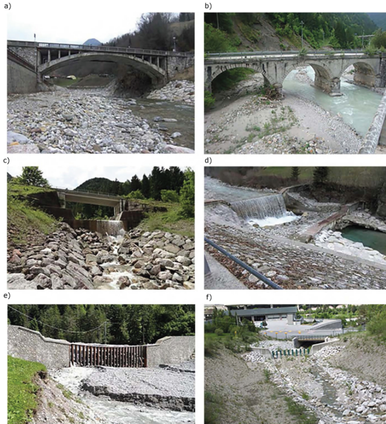
Figure 3. Photo record of the structures inspected: (a) upstream view of Bridge-1: Pretest and Test-1. (b) Upstream view of Bridge-2: Test-2. (c) Upstream view of Bridge-3: Test-3. (d) Check dam-1: Pre-test and Test-1. (e) Opening of Check dam-2: Test-2. (f) Upstream to downstream view of Check dam-3: Test-3.
