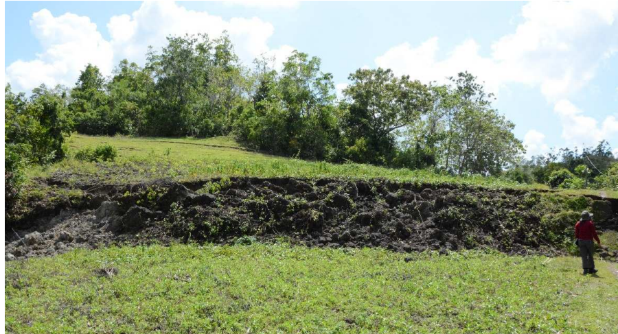
Fig. 4. Formerly gently sloping ground split through reverse faulting into an upthrown block and lower block forming a 3 m high wall that extends for several kilometers. Photo: AMF Lagmay.
