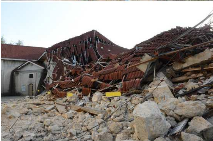
Fig. 2. Images of the disaster: (A) collapsed house in Sagbayan municipality, Bohol. (B) Inabanga church in Bohol. Photos: AMF Lagmay.
