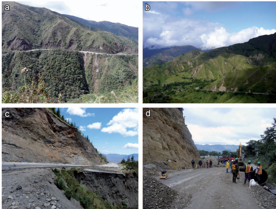
Fig. 2. Landslides occurring along the investigated highways. (a) Typical landslides of the wet metamorphic part of the study area in the east. (b) Typical landslides of the semi-arid, conglomeratic part of the study area in the west. (c) highway destroyed by landsliding. (d) A highway is cleared from a recent landslide occurrence.
