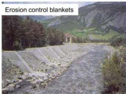
Fig. 7. Some structural measures to cope with flash floods in the Barcelonnette area.
