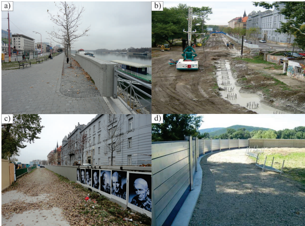
Fig. 5. Various structural flood protection measures in the city of Bratislava, see Table 1 ; (a) concrete wall, (b) underground sealing wall, (c) reinforced concrete wall, (d) mobile flood wall.
