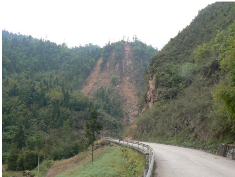
(b) Shallow slope failures (photo taken by Dr. M.M. Wang)
