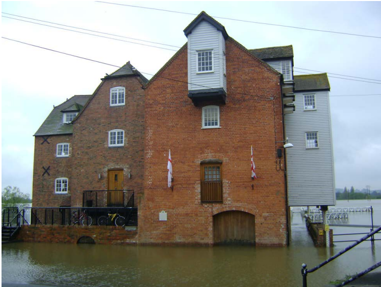
Fig. 1. Recent flooding at Tewkesbury (Stephenson and D’Ayala, 2012).
