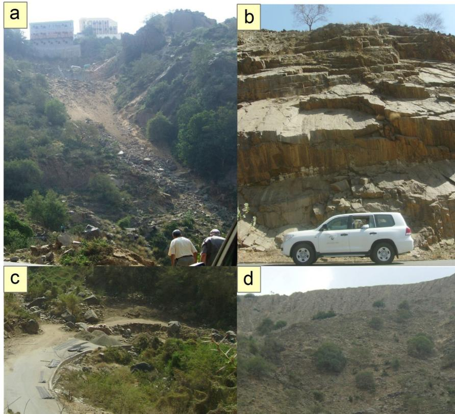
**Fig. 4.** Field photographs taken throughout field trips one and two: **(a)** landslide caused by debris flows within an ephemeral valley; **(b)** area prone to landslide development by failure along fracture planes that dip towards the road; **(c)** intersection of debris flow with road; and **(d)** landslide caused by debris flow related to overland flow, where features indicative of overland flow include the presence of rills and loose rock units of various sizes on the slopes.
