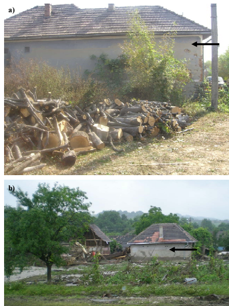
Fig. 6. The flash-floods marks in the affected areas: (a) Lupeni village – Feernic basin; (b) Uioara de Jos village – Ciunga basin.
