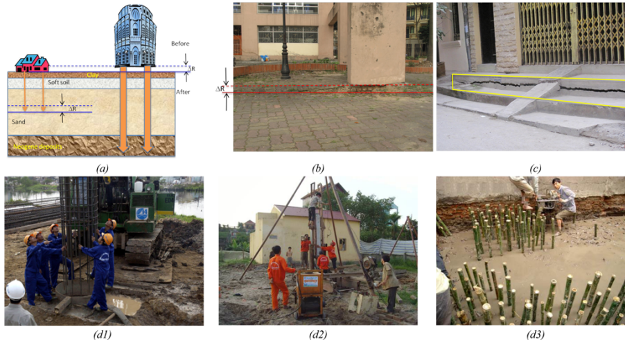
Fig. 10. (a) Model of subsidence process. Example of subsidence damages in (b) Dinh Cong residential zone at Hoang Mai subsidence area. (c) Van Quan residential zone at Ha Dong-Thanh Xuan subsidence area. For location of investigation points, refer to Fig. 3. Several type of foundation is using in study area: (d1) auger-cast piles, (d2) concrete pillars, (d3) bamboo piles. Photo: http://www.cocbetong.vn .
