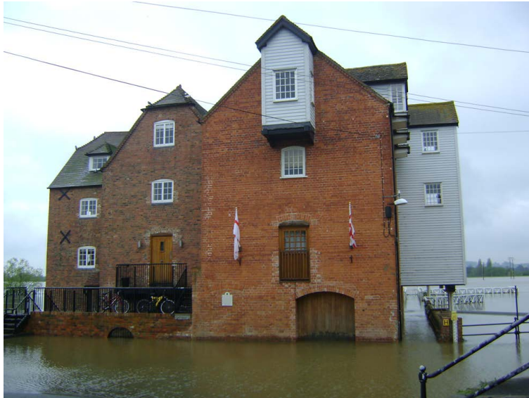
Fig. 1. Recent flooding at Tewkesbury (Stephenson and D’Ayala, 2012).
