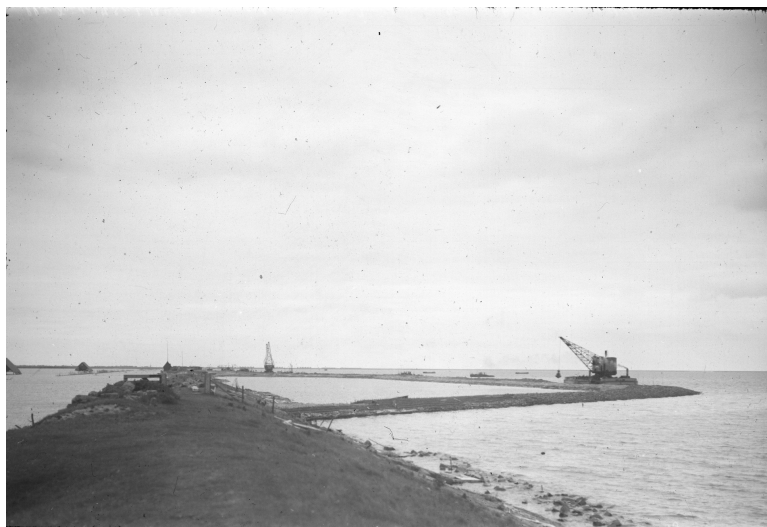
Fig. 7. Reconstruction works around the breach in August 1945. The polder is on the left with some roofs of farm houses visible in this picture and Lake IJssel is on the right.
