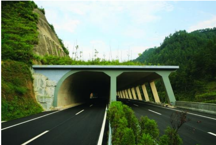
Fig. 1. Rock-shed with reinforced concrete columns, foundation and a roof slab.
