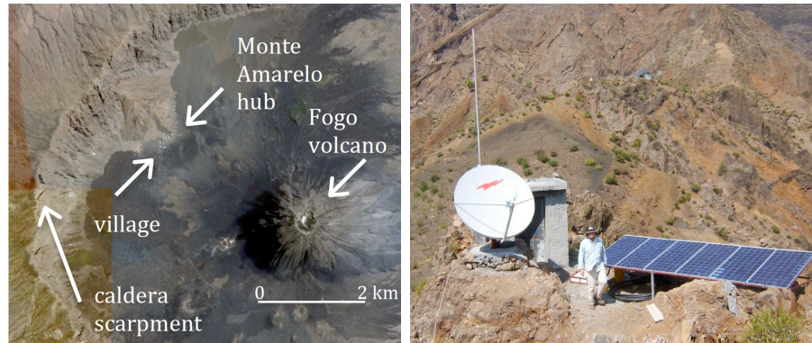
Fig. 5. The VSAT station in Fogo volcano’s caldera. Left: Google Earth view, showing Fogo volcano, the caldera scarpment and the site of the Monte Amarelo hub. Right: setting up the satellite antenna and power supply. The mast behind the dish will receive the antennas of the local links.
