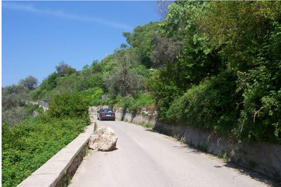
Fig. 20. A limestone block fell on Kruja urban area during heavy rain on 2010.
