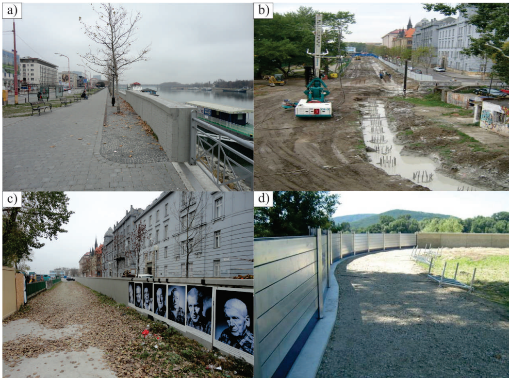
Fig. 5. Various structural flood protection measures in the city of Bratislava; (a) concrete wall, (b) underground sealing wall, (c) reinforced concrete wall, (d) mobile flood wall.
