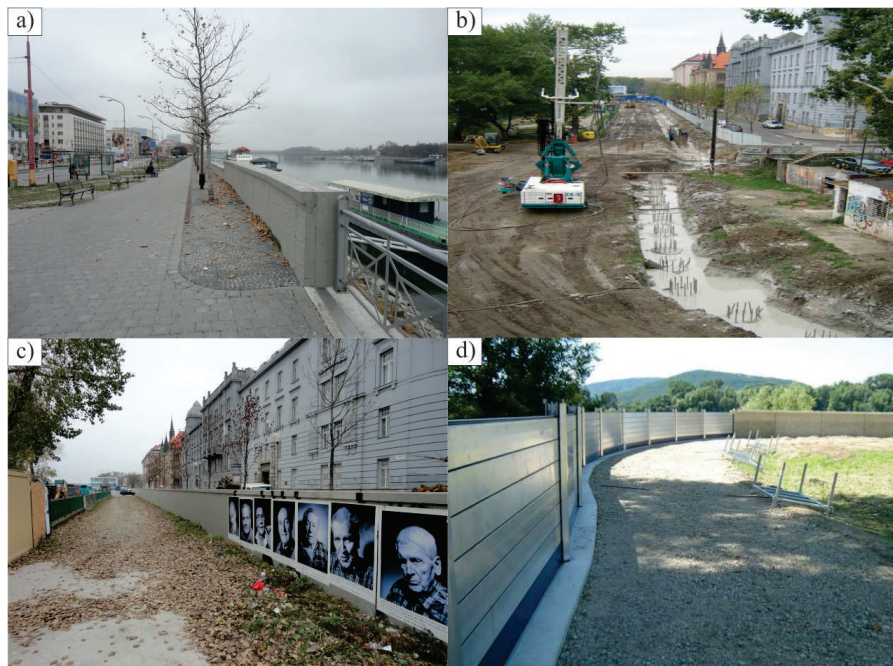
Fig. 5. Various structural flood protection measures in the city of Bratislava; (a) concrete wall, (b) underground sealing wall, (c) reinforced concrete wall, (d) mobile flood wall.
